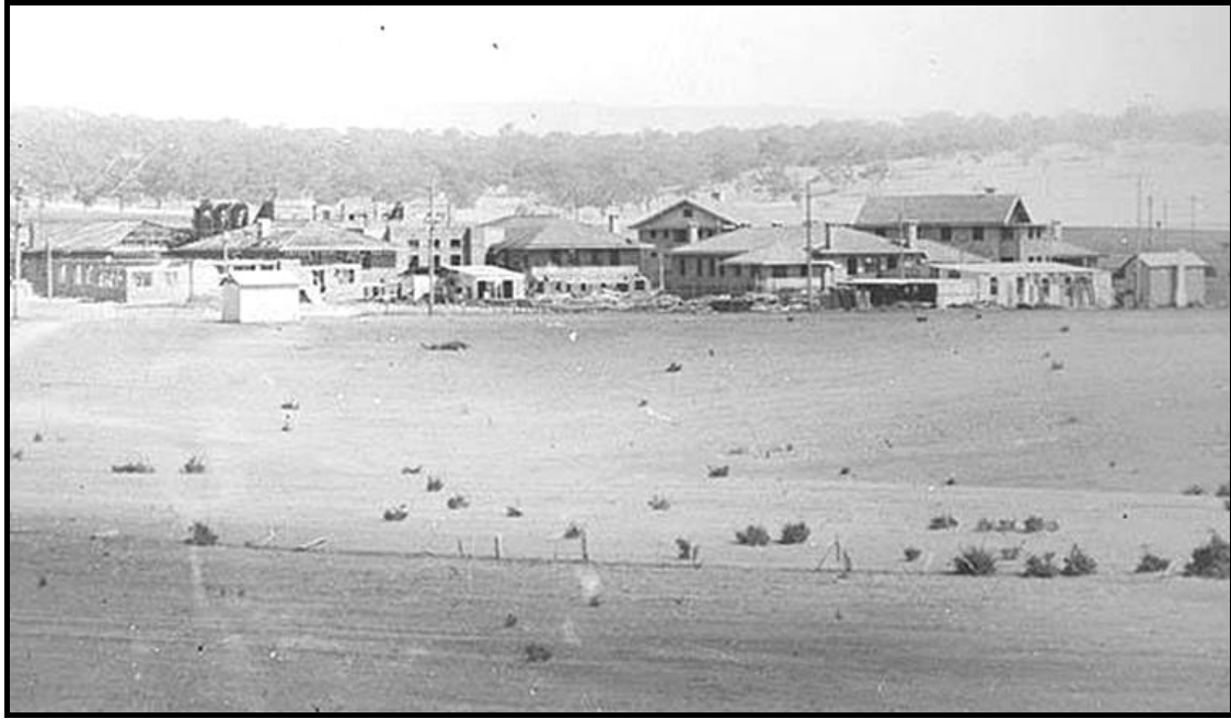
Above – Hotel Canberra under construction 1925. This hotel was Hostel No 1 – the politicians’ hostel and was the first erected in the territory. It was followed by the Hotel Kurrajong in 1925. In 1927 the Hotels, Acton, Ainslie, Wellington opened followed by the Hotel Kingston and later in the early 1930s the Hotel Civic. The Rex Hotel in Northbourne Avenue was built after World War 2.
