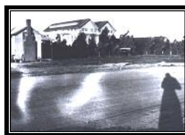
Photograph bottom of page – left side column : On the left is the Engineers' Mess and on right – the Power House. The photograph was taken circa 1926 by Jack Benson (shadow) who also lived at the Mess before marrying. The road is Wentworth Avenue.
