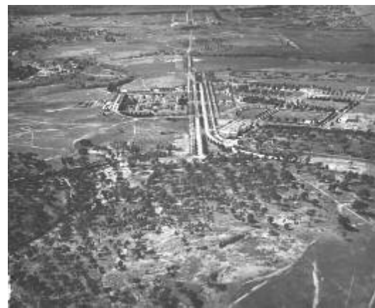
Above Capitol Hill, Commonwealth Avenue and off to left Hotel Canberra circa 1927 and below – two photographs of Hotel Canberra.
