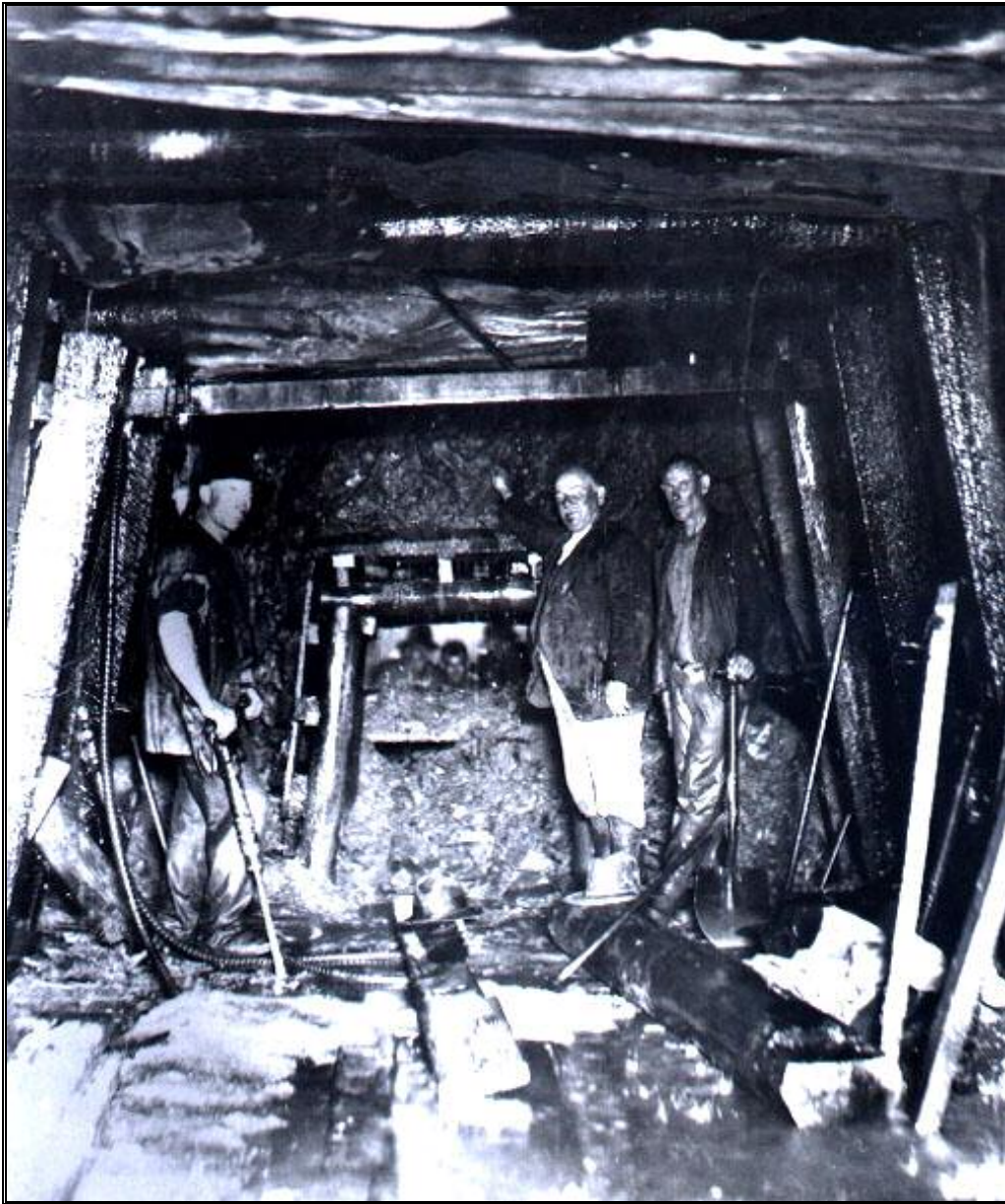
Above: Jeremiah Dillon (the only one not wet) in one of the tunnels. The photograph is one of the Mildenhall Collection in Australian Archives Canberra. At times the sewer men had to work in water up to their waists. In the centre are the faces of men in the other section of the tunnel. Jerry Dillon started work on the sewer from 1915. He also was put off in 1916 when work stopped. Following the resumption of work in 1921 he again took up the position of Foreman of the Sewer Works. He died in 1929. Between 1922 and the time of his death he lived in a small brick cottage in Hutchins Street - now opposite the Yarralumla Shops. It is in Section 64 and has little changed from the time that Jeremiah and his wife lived there.
