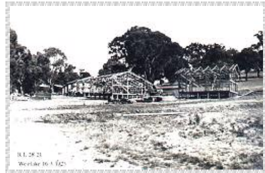
The above photograph was taken in 1924. The unfinished cottage on the right is 27 Westlake where my family lived from 1941 until 1959. These cottages were sold and moved to new sites from the mid 1950s. The last cottage was moved in 1965. The site of the majority of these cottages today is Stirling Park in the Canberra suburb of Yarralumla. The sites of cottages 22-62 are in Stirling Park and the sites of 1-20 are now in the grounds of the Mexican Embassy in Yarralumla.
